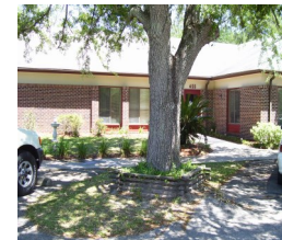
Outside view of a 64 person ICF/IID facility.
