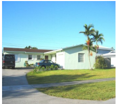
Outside view of a 6 person ICF/IID Facility.
